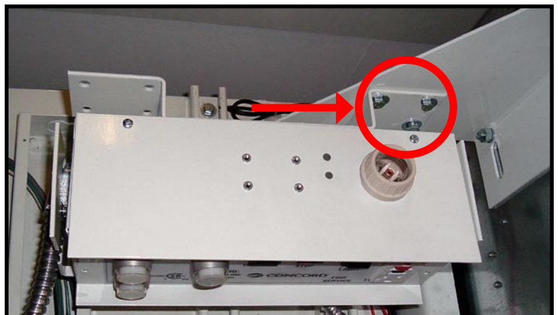
Figure 91 CTIS mounted, top view
