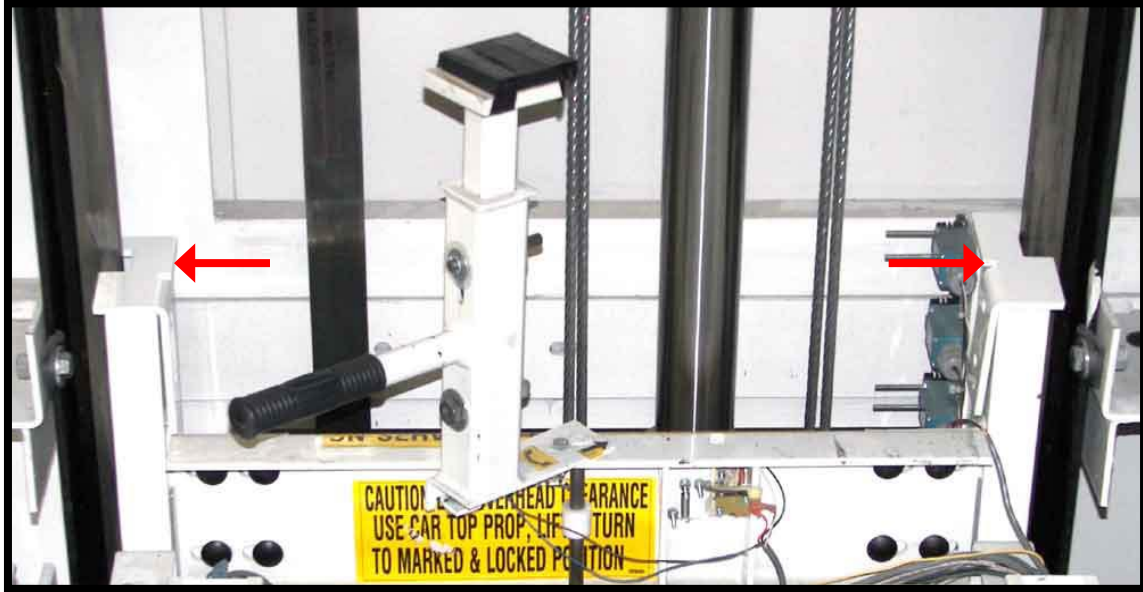
Figure 40 Stile Retainer Installation
