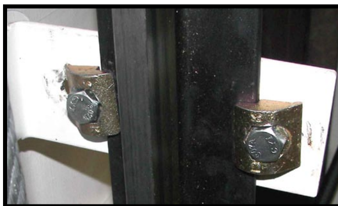
Figure 19 Rail Clips on Rail
