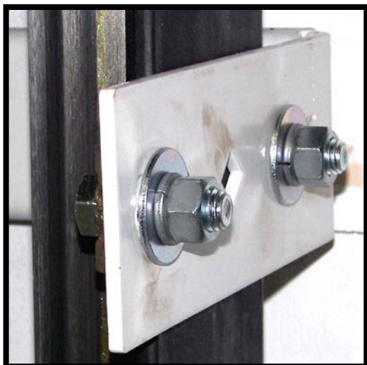
Figure 18 Rail Clips on Leaf Bracket
